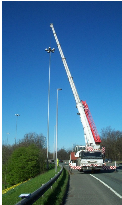
Replacement of high mast lighting with conventional lighting
